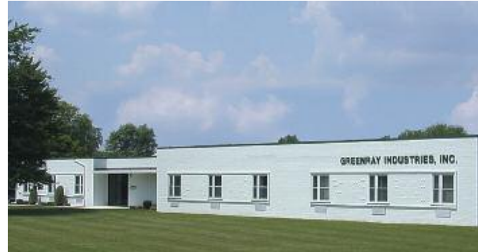
Greenray Industries, Mechanicsburg, PA
